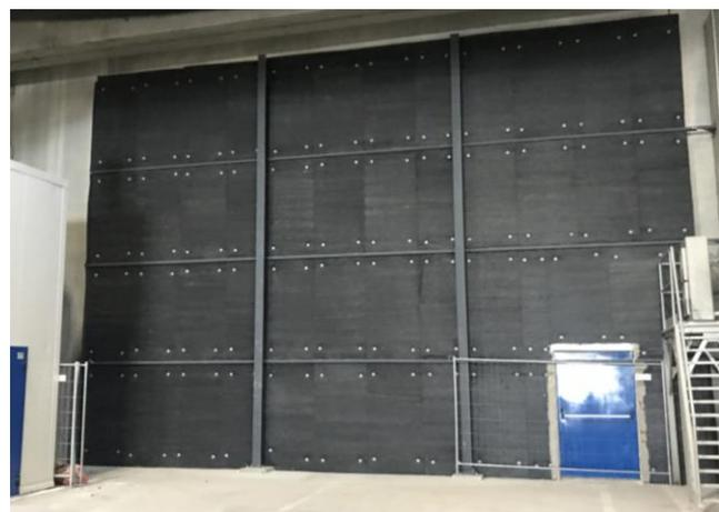
Fig. 2 - rivestimento pareti tunnel box
